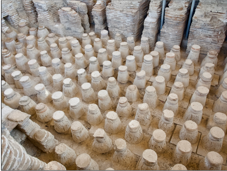
A bath house that includes 3 rooms (1) hot room or sauna (2) cold room (3) cool room for transition from sauna to cold. Note the remains of pillars made of mud bricks that were used to lift up the floor. Slaves would burn wood outside through arches to heat the sauna. This was a very large structure. (June 2022)
